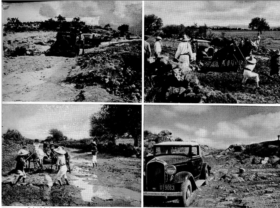
Fig. 2. The Pan American Highway on the way to Mexico City under construction c.1932. Source: Franck and Lanks, 1940.
